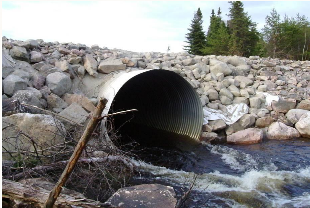
Installation de ponceaux conformes
